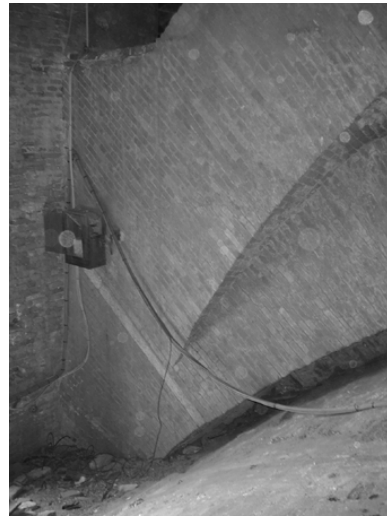
Fig. 7. Detail at the intersection of the two oblique planes of the arches
