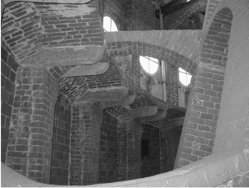
Fig. 9. Catwalk of the dome supported by granite corbels connected to the relieving arches
