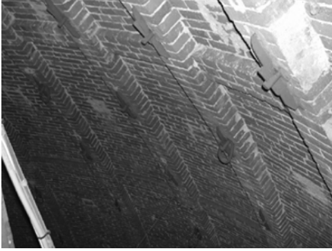
Fig.12. Ribs and supporting system of the external covering in stone slabs
