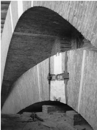
Fig. 6. Oblique arches that support the dome showing the stone blocks that stiffen them.
